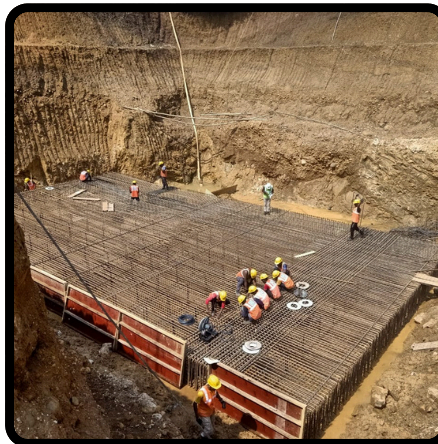
Sump house raft foundation work kpil jashipur, odisha
